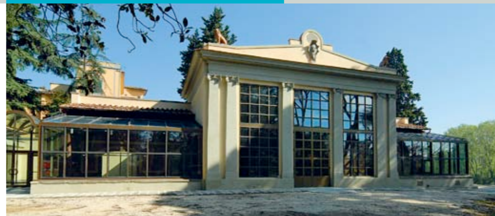
The front glazings could also be restored to their original look with the Forster thermfix vario pillar/bolt system with its slim sightline of 45 mm.
