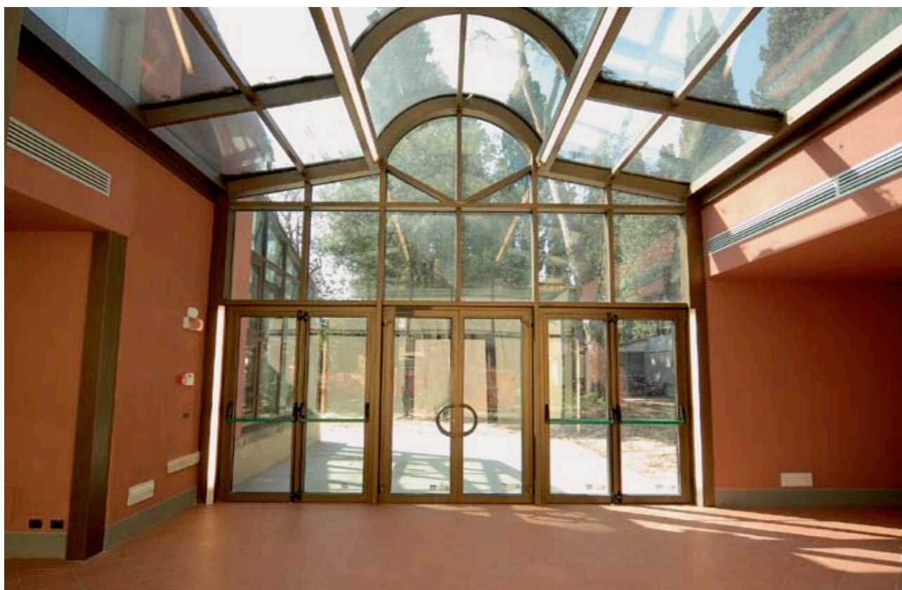
A particular challenge for the construction engineers – the curved roof glazing structure.
