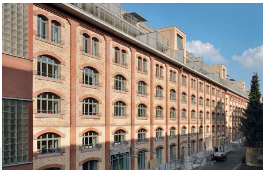
Filled with new life: the warehouse at Giesshübelstrasse 62 in Zurich.
