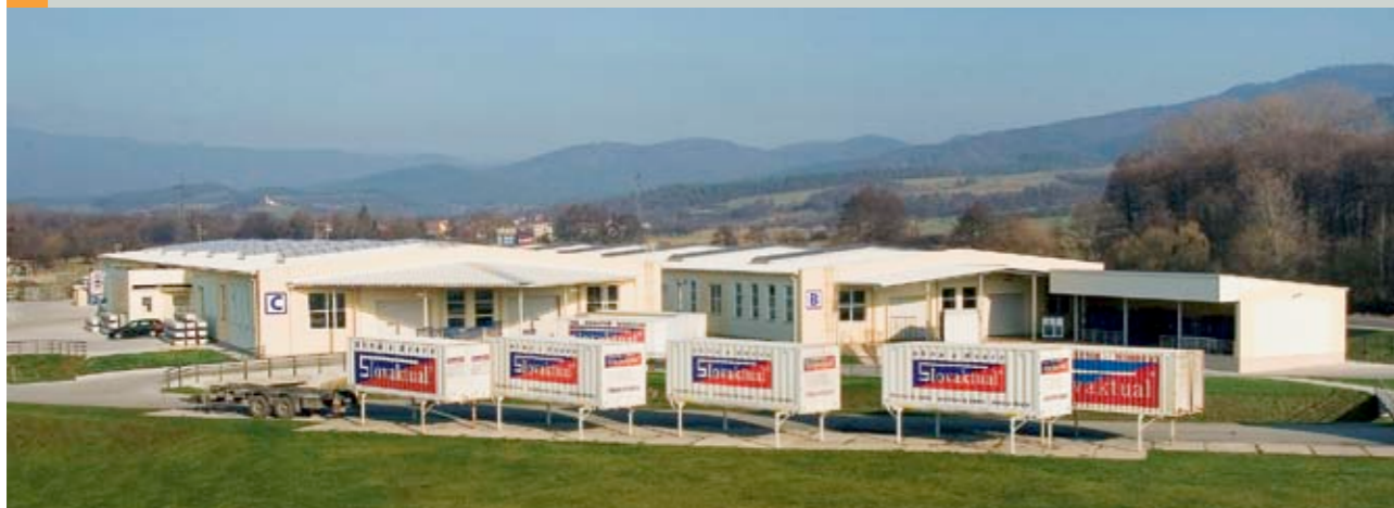
Windows are manufactured in 22 colour combinations in halls B and C.
