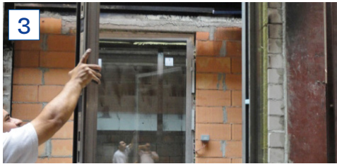
Mount door leaf, align for air gap.
