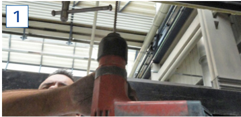
Fix door frame at the top end.
