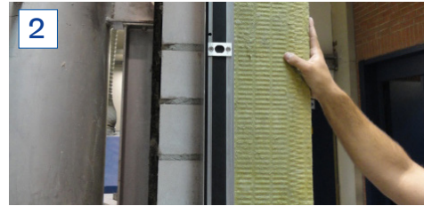
Fill (and close) joints.
