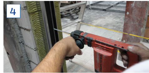
Drill lateral anchor holes.
